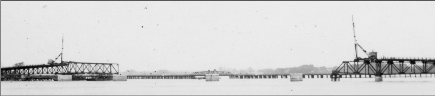
Main span of 275 feet, vertical clearance of 40 feet, continuous unit of 675 feet, length over all of 1,528 feet
