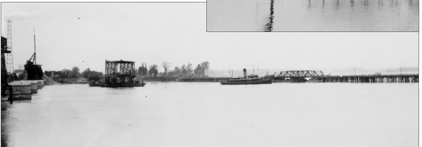
Floating in a new section on two barges. The coal-fired "Mitchell Davis" tugboat is in the middle of the two photos below and to the right. The swing draw in the old railroad bridge can easily be seen at the tug's bow in the bottom photo.
